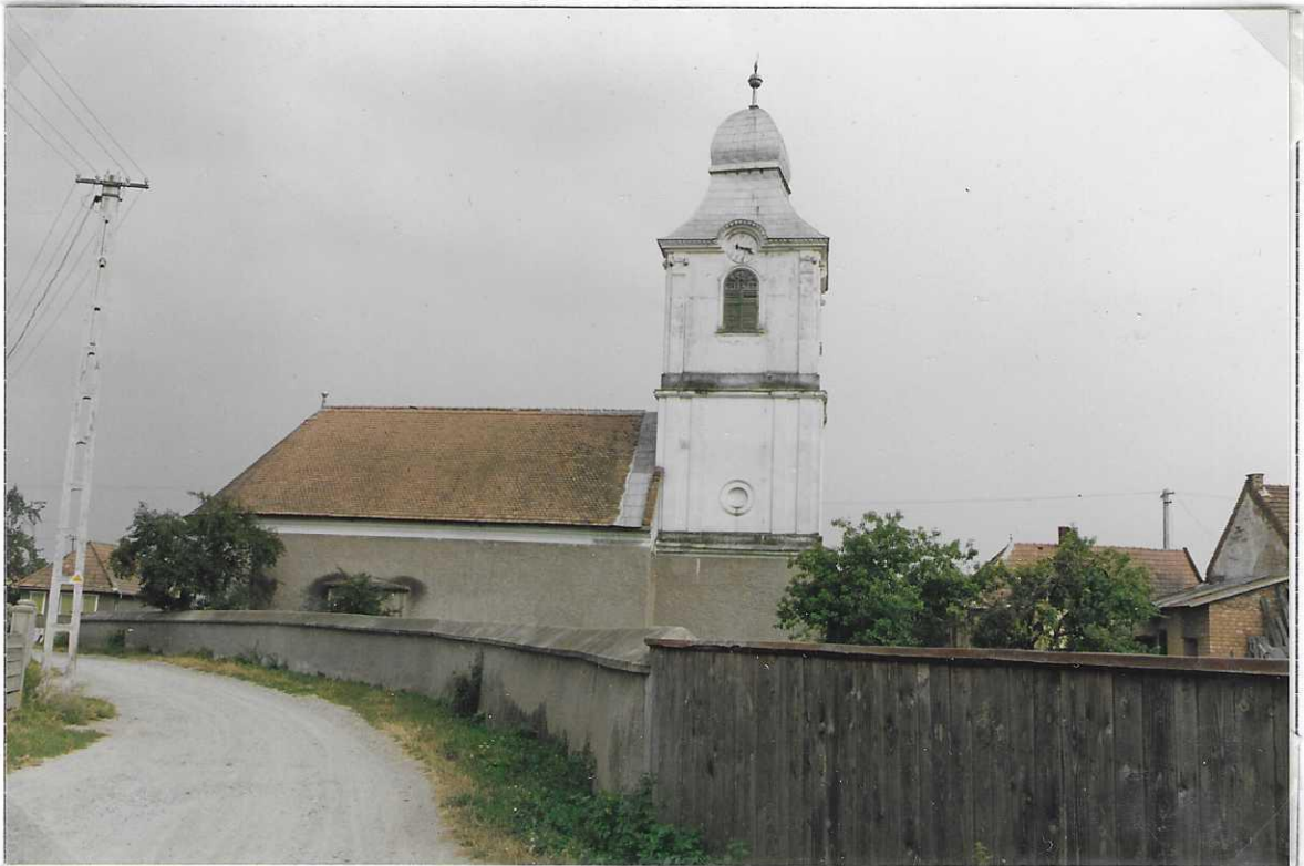
View of the church from the rear
