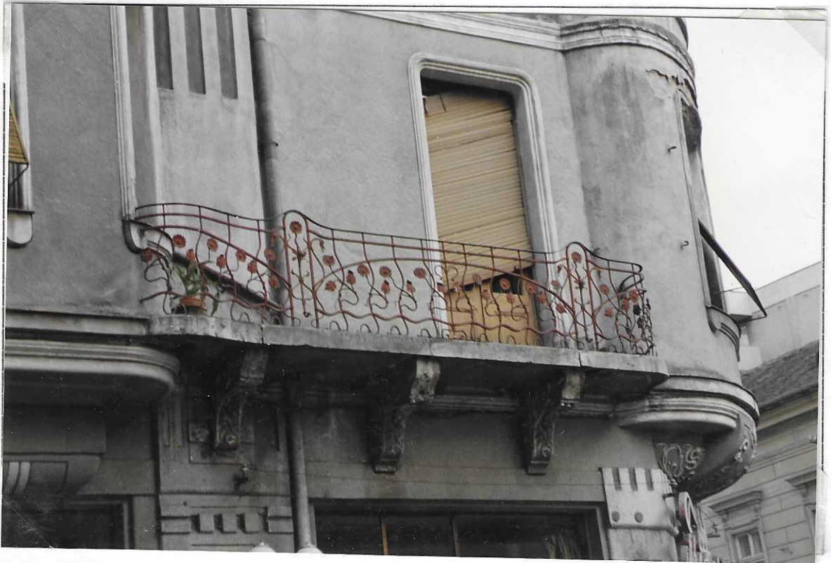
Closeup of balcony railing
